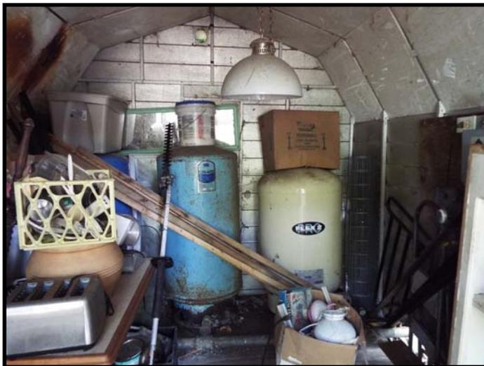
**The pump house includes the pressure tanks for the system and the well head is outside . This appears to be a 4 inch well. Owner had a new submersible pump installed about 3 years ago.**
