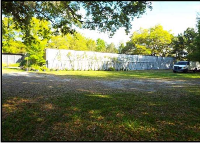
**80 x 95' Shade house that does not have the height of the larger house. Also steel construction with poly roof.**
